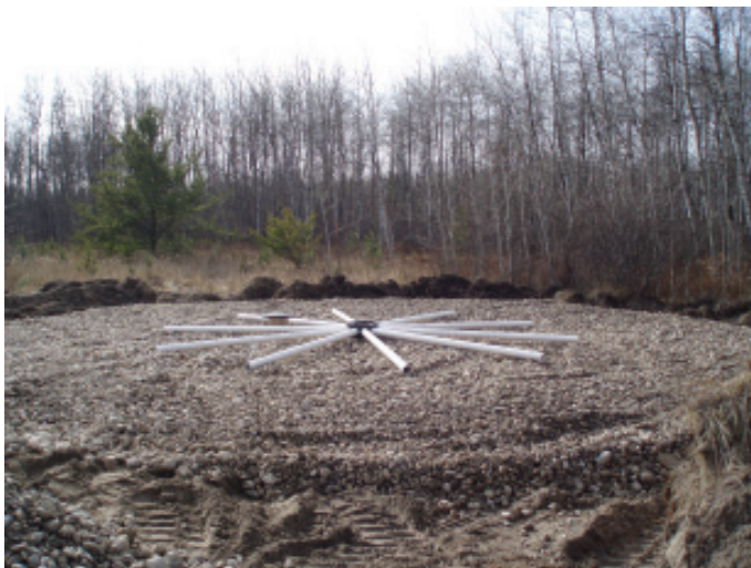
Installation of a septic field.
